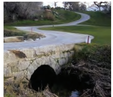
One of 12 Bridges
