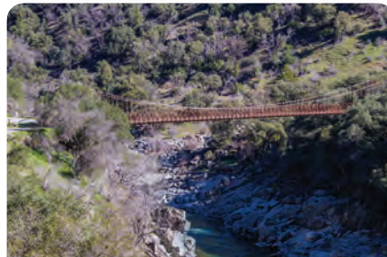
Yankee Jims Bridge
