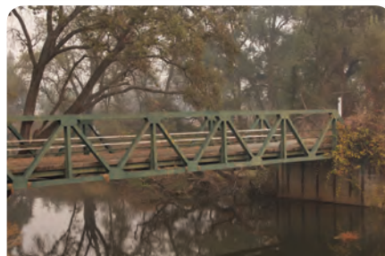
Coon Creek Bridge
