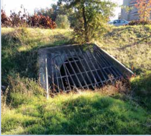
Culvert Bridge in Mansion Oaks
