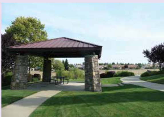
A second Orchard Creek North Trail entry leads from this personal park in Village 26B/C at the end of Emerald Lane (see trail at right). All Open Space names are posted; note their names and carry your cell phone should an emergency arise
