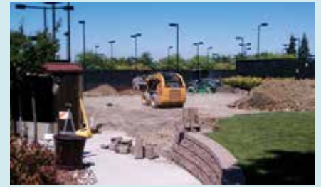
The three new pickleball courts are under construction
