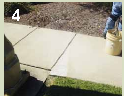
Hazardous, mismatched sidewalk sections like the one in photo 1 are repaired by grinding them to smoothness (photos 2 & 3) so they are level as in photo 4
