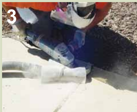
Hazardous, mismatched sidewalk sections like the one in photo 1 are repaired by grinding them to smoothness (photos 2 & 3) so they are level as in photo 4
