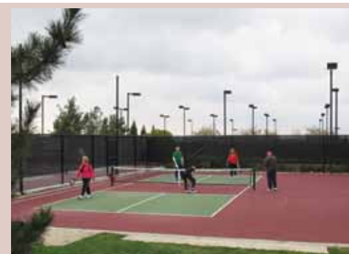
New Pickleball Court in use for a tournament in December. Improvements include fencing, a gate to access the three original courts, additional lighting
